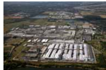
Completion of power sourcing for Neuss smelter
